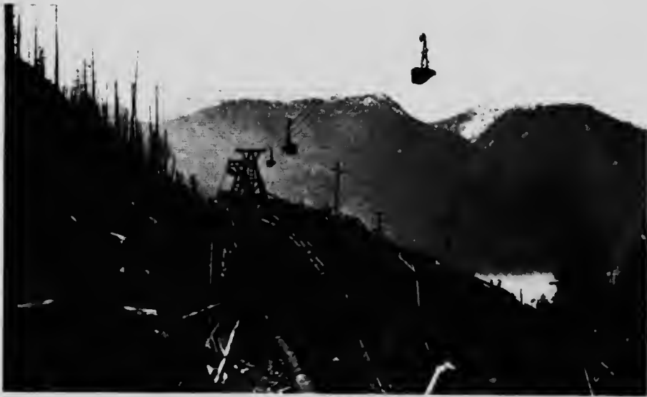
Britannia Mining and Smelting Company Limited. Aerial Tramway conveying Ore from Britannia Mine to the Mills at Britannia Beach. Howe Sound is seen on the right of the picture.
